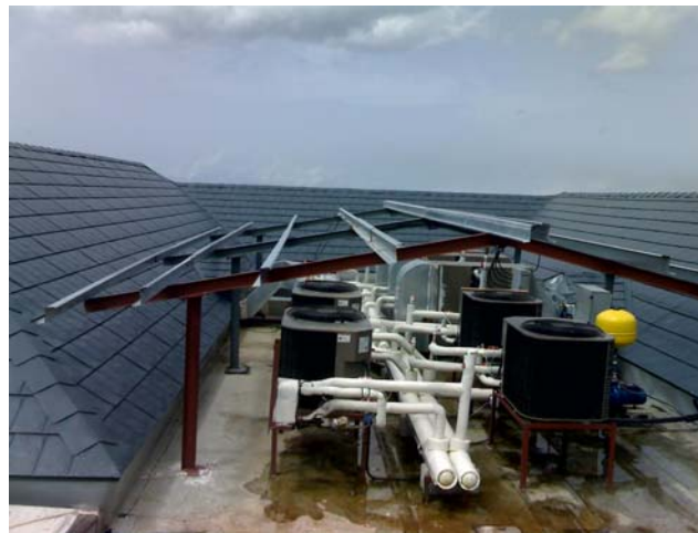
Fig. 5 – High Efficiency Mini Chiller with Heat Recovery
