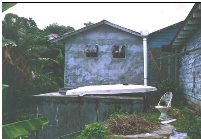
Figure 2.25 - Rainwater catchment system. Rainwater is collected from the roof of this back-of-house building to supply water to the laundry. The large-diameter downspout conveys the water from the roof's gutter to the concrete storage tank.
