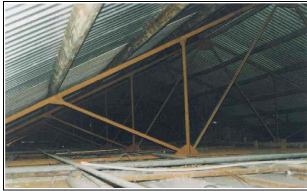
Figure 2.41 - This attic of a Jamaican hotel has no insulation or radiant barrier. Heat from the metal roof is radiated directly onto the gypsum-board ceilings and into the rooms below.
