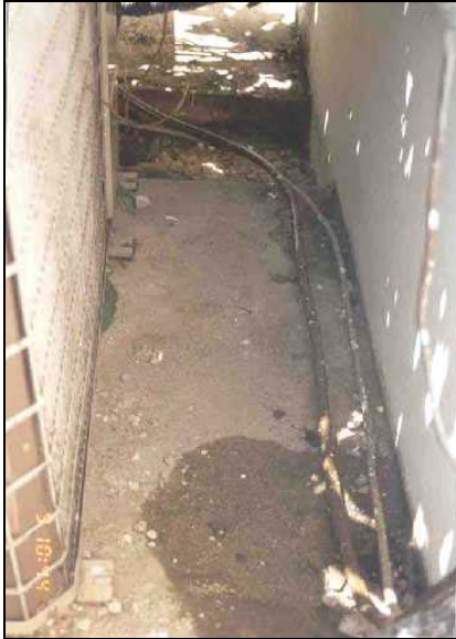
Figure 2.46 - Bare refrigerant line connecting the condenser to the evaporator of a mini-split a/c system.
