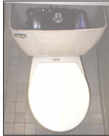
Figure 2.20 - Pressurized-flush toilet (tank cover has been removed to show the pressurization system).
