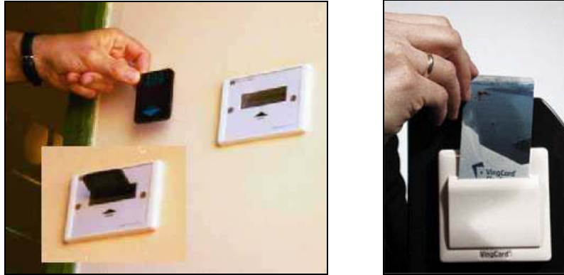
Figure 2.43 - Card-activated energy-saver switches that are used to control the operation of guestroom a/c systems and lights.
