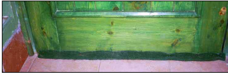
Figure 2.38 - Low cost door sweep made from a strip of felt material.
