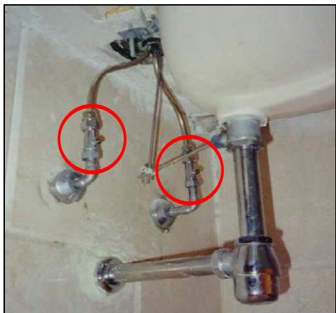
Figure 2.13 -Typical faucet shut-off valves.
