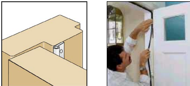
Figure 2.36 - Nail-on weather-stripping (left) and tape-on weather-stripping (right).
