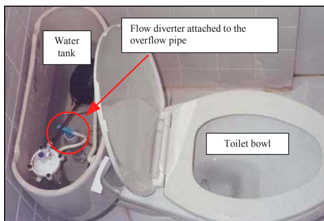
Figure 2.24 - Flow diverter installed on a gravity-flush toilet.
