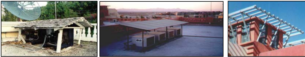
Figure 1.5 - Examples of condenser shading options used in hotels.
