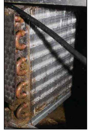
Figure 2.45 - Condenser coils of a refrigerated kitchen cabinet before and after cleaning.
