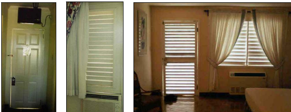
Figure 2.34 - Typical air infiltration problems in air conditioned areas: gaps around doors and through-the-wall a/c units, gaps between the slats of louvered windows, and fixed open louvers on doors.
