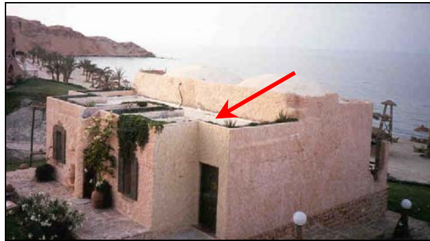
Figure 2.39 - Reflective paint applied to this roof reduces the roof temperature and associated solar heat gains into the spaces below.
