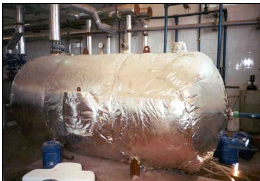
Figure 2.51 -Example of a well-insulated hot water storage tank.
