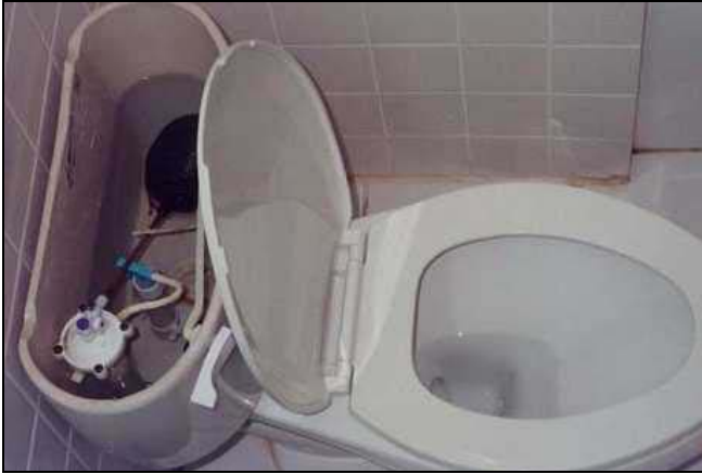
Figure 2.19 - Gravity-flush toilet (tank cover has been removed to show the components of the flush mechanism).
