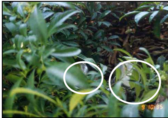
Figure 2.27 - These two light fixtures are completely covered with overgrown vegetation. Other than creating a unique “burning bush” effect, these lights no longer serve any useful purpose.
