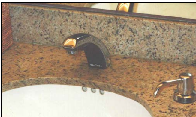
Figure 2.15 - Touch-free metering faucet installed in a public bathroom.
