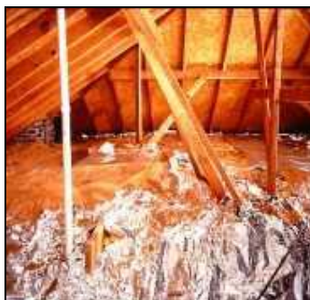
Figure 2.40 - Radiant barrier installed on an attic floor.
