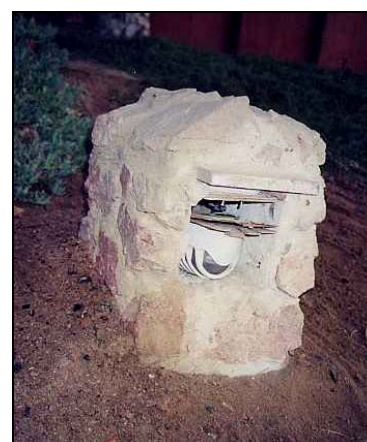
Figure 2.26 - An extreme example of a poorly designed light fixture: A 40-Watt bulb is first covered by a frosted lens and a thick protective mesh; the whole fixture is then placed upside down in a narrow alcove cut in a stone pillar.
